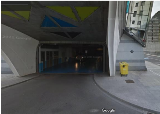
Figure 31 Mechanical entry Source: Google Maps "street view."
