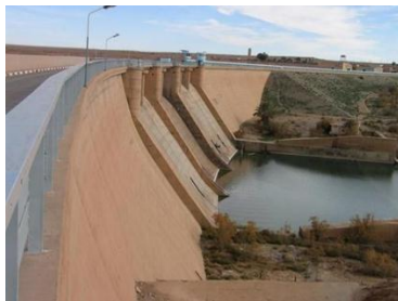
Figure 45 : Barrage djorf torba
