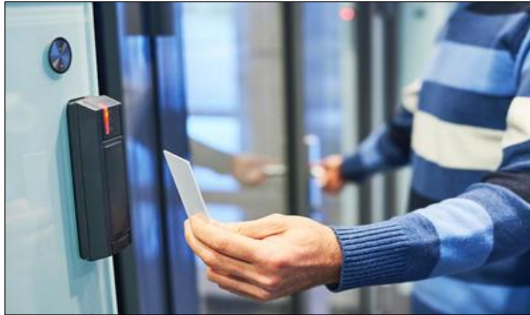
Figure 1 Access control using an electronic door [4].
