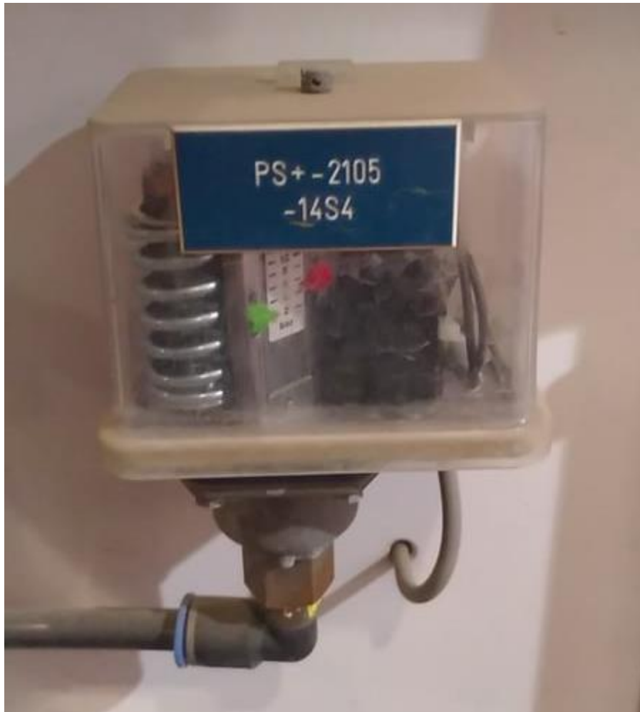
Figure II.14 : Pressostat
