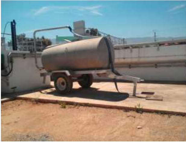
Figure III.6: Stockage des graisses
