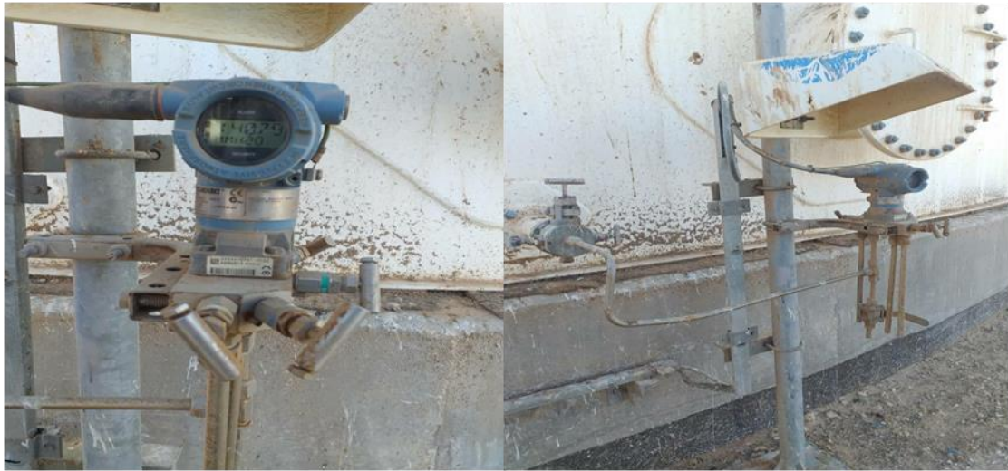
Figure 1.8 Transmetteur de pression.
