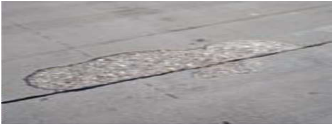
Figure I. 29: Ecaillage [2].
