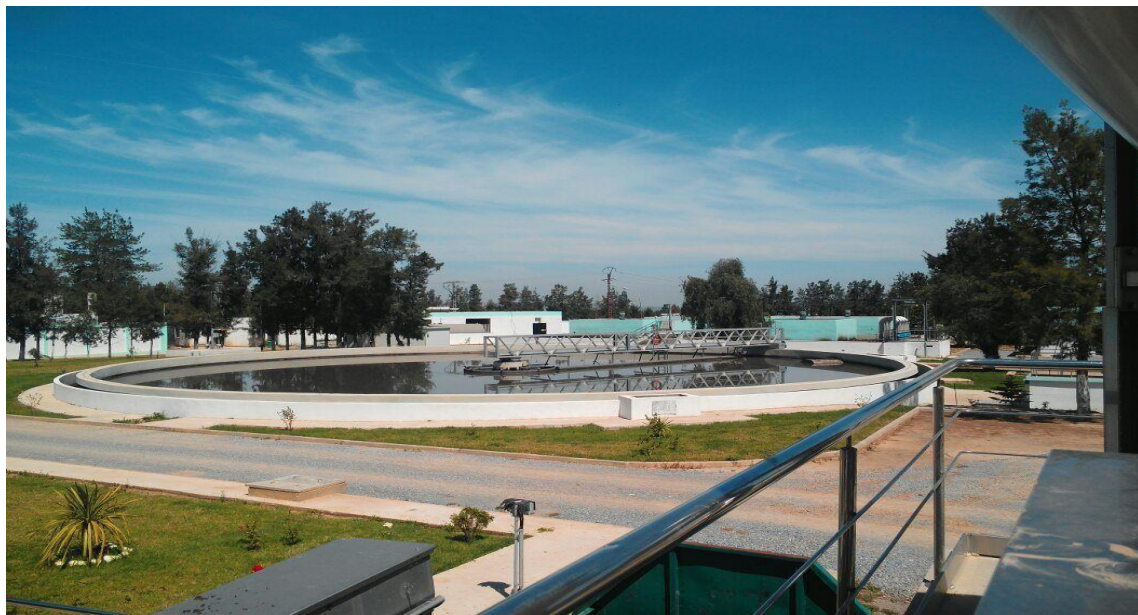
Figure 1: Station d'épuration de Béni Mered (Photo originale)
