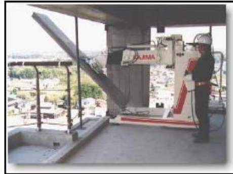
Figure I.26: Robot de construction
