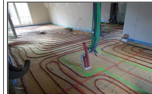
Figure II.66: Planchers chauffants Source : http://www.actuarchi.com/2011/03/26-logements-bbc-tourcoing-atelier
