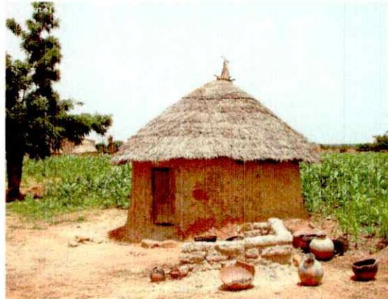
FIGURE 15 PHOTO D'UNE HUT FAITE EN TERRE CRUE.
