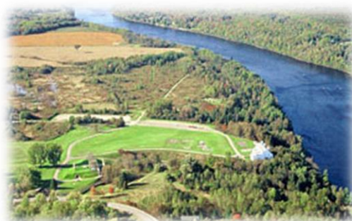
Figure 21: Forges-du-saint Maurice Québec Canada.
