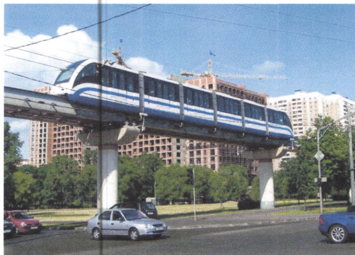
Figure 44 : poteau monorail Source : Igor F, 2007
