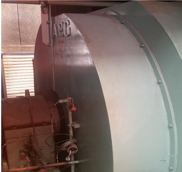
Figure 2.15: alternateur.
