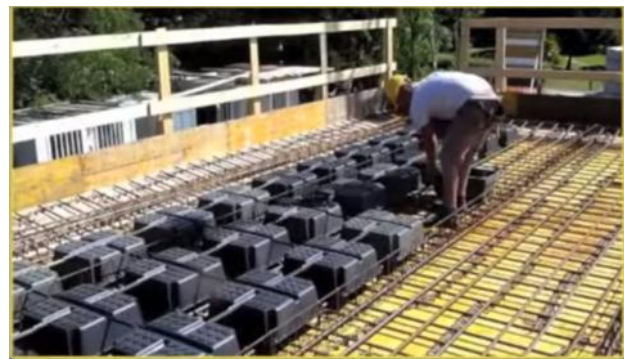
Figure 66: plancher allégé U-boot béton Source: Persello .(2005)
