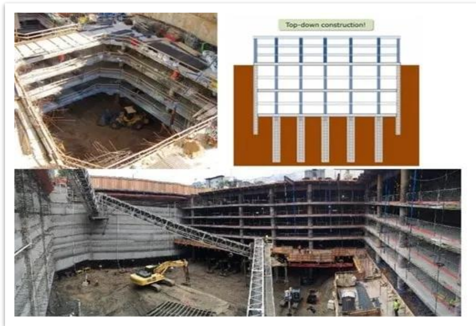
Figure I. 7 : Construction de type "Top Down". [1]
