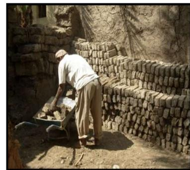
Fig.2.20. Assemblage de la pierre sree : Gourna a tale for two villages
