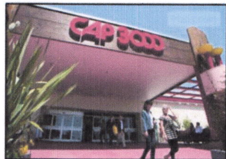
Figure IV-35 : Centre commerciale Cap 3000 Nice France
