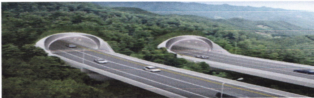
Figure II-8 tunnel de Texenna. Source : http://www.jijel.info
