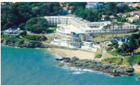
Figure 60: L'hôtel Alliance Thalasso & SPA Pornic/ France
