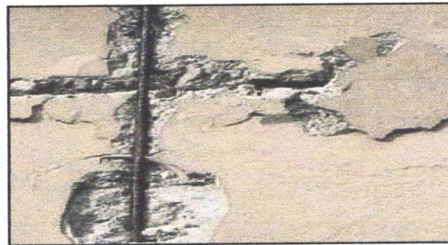
Figure 22 :La corrosion source : www.wikipedia.com
