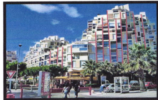
Figure 42 Pare –soleil verticaux
