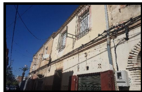
Figure 22 : La façade Principale.
