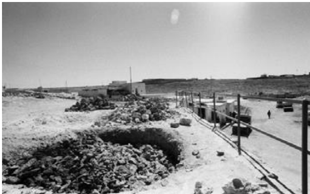
Figure36: Phase de construction
