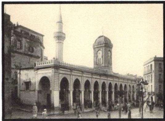
Photo 3.1: mosquee Salah bay
