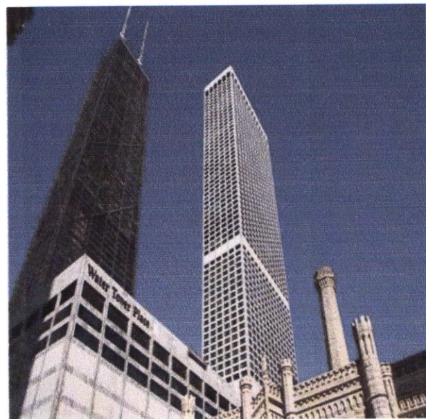
Figure 24: Centre d'affaires Water Tower Place
