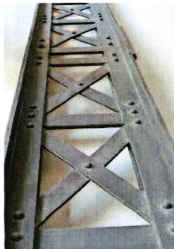
Figure 81: treillis riveté
