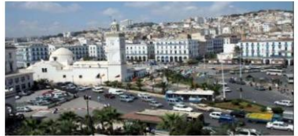
Figure 25; Immeuble mixte, place des martyrs (Google image)
