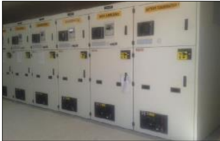
Figure I.15 I.5 Tableaux MT
