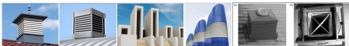
Fig.97. Modern passive stack ventilation terminals; Suncatcher and windcatcher. (a) External view of slots and of sun pipes for a suncatcher and (b) The four air flow segments of a windcatcher.
