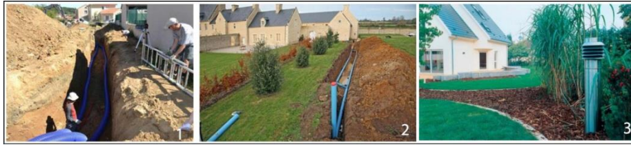
Fig.66. Installation a Canadian well.(Source: Google image)
