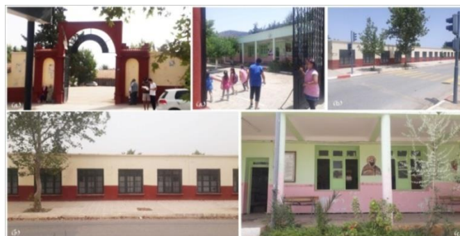
Fig.106. Views of different parts of the school; main entrance(a); Southern facade view (b); Northern wall of classrooms bar (c).
