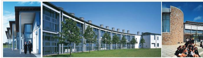
Fig.6. Different views show the wind tower of the HAUTE VALLE school.
