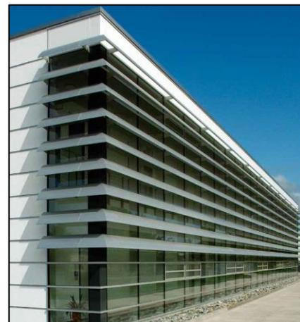
**Figure III-86 :** Lames brise soleils en aluminium.
