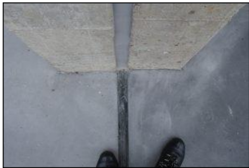
Figure 95 : joint de dilatation.
