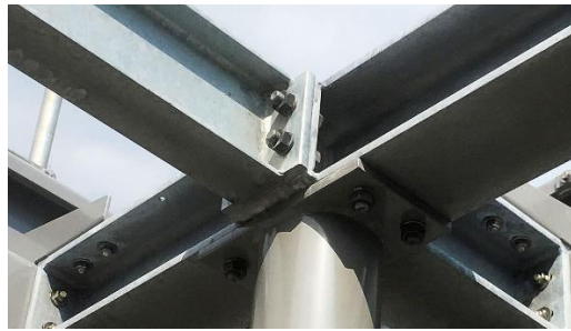
Figure I.4 : Assemblage boulonner.
