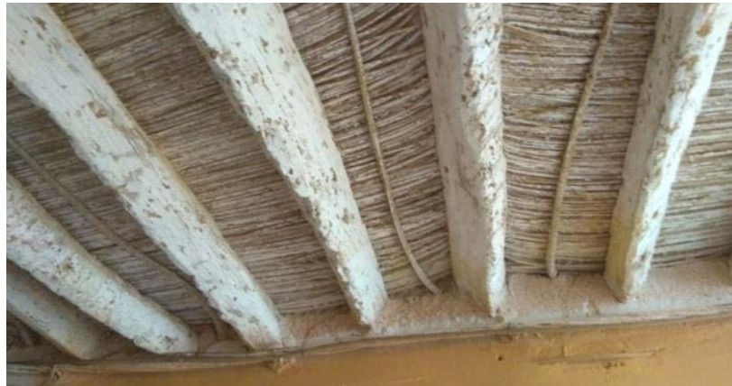
Figure I.30: Floor of a reed-covered passageway in the Ksar of Al Atteuf [71]
