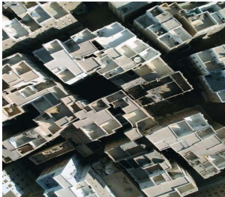
Figure I.5: (a) Terrace houses in the town of Shibam [16]
