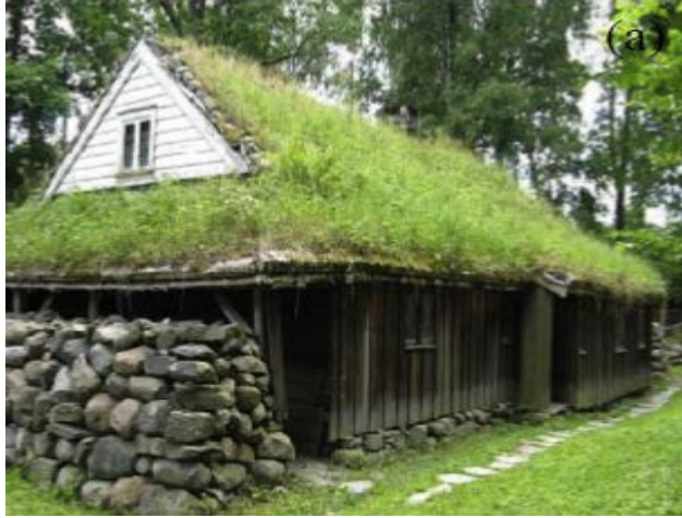
Figure I.16: Buildings with green roofs: (a) Traditional sloping green roof with vegetation in Norway [42]
