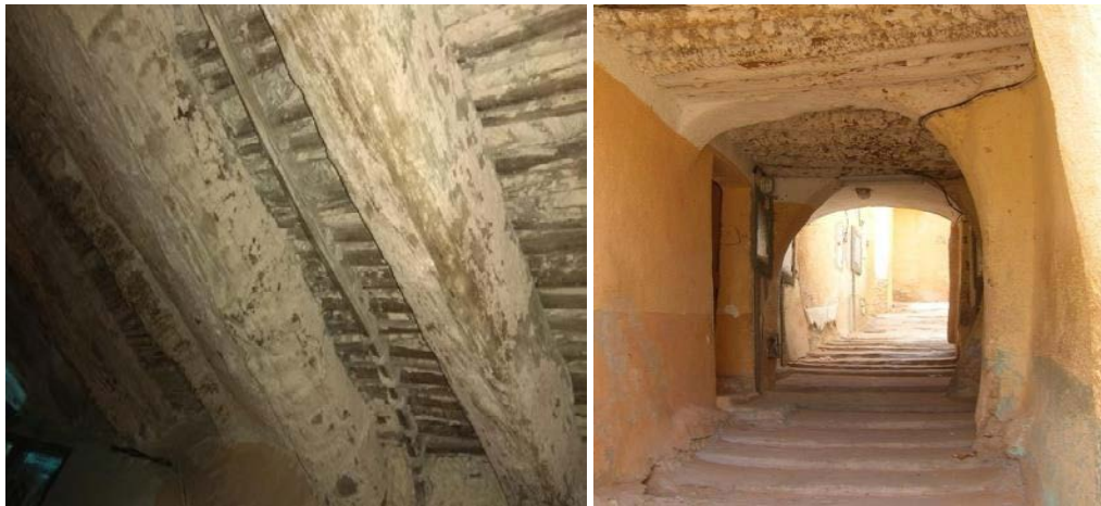
Figure I.27: Photos of a floor made of palm trunks and branches in a covered passageway of the Ksar: (a) floor in a passageway of the Ksar Al-Atteuf; (b) floor in a passageway of the Ksar of Béni Isguen [1]
