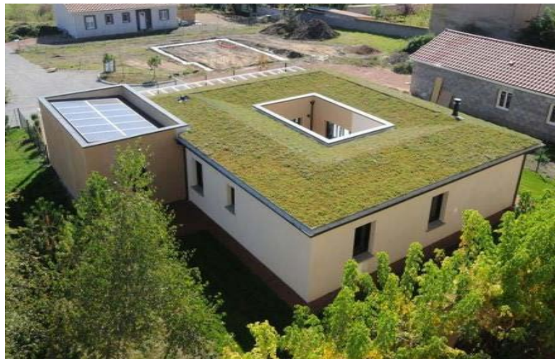
Figure I.16: Buildings with green roofs: (b) flat green roofs and rounded green roofs respectively [43]
