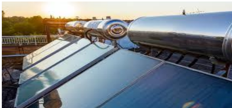
Figure III.1 : chauffe-eau solaire plan. [13]
