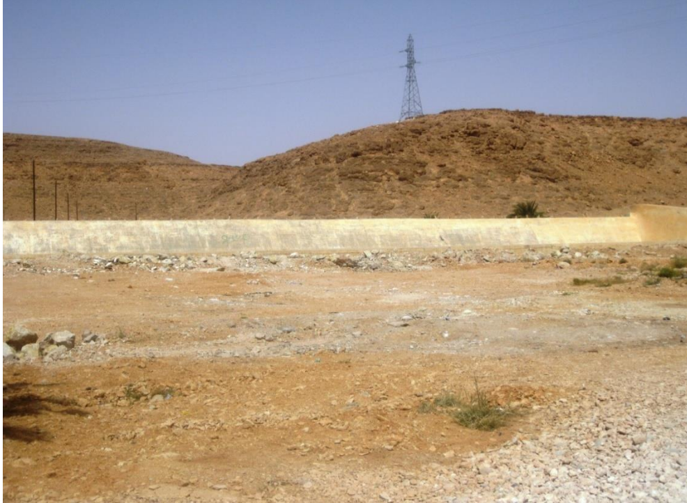
Fig.2.1. barrage Ahbess Ajdid
