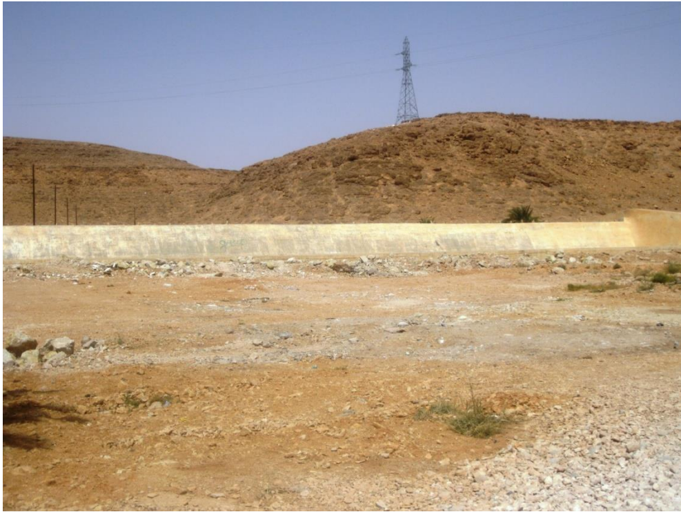
Fig.2.1. barrage Ahbess Ajdid
