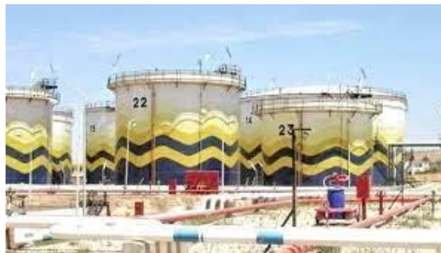
Figure 1-4 Stockage des carburants.[6]
