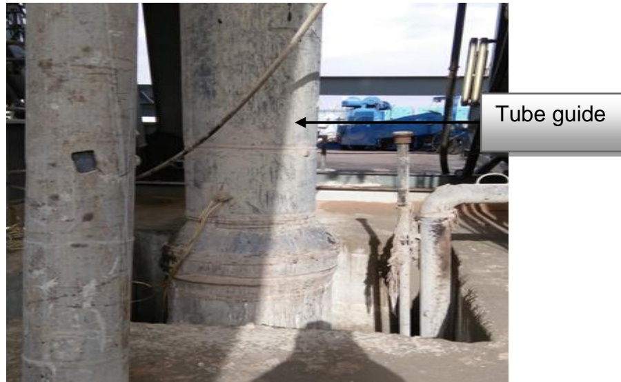
Figure 02 : Le tube guide.
