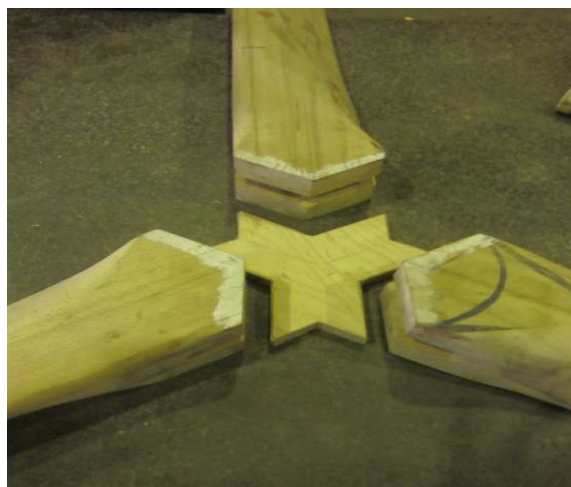
Figure IV-C-3 : La plaque a collée
