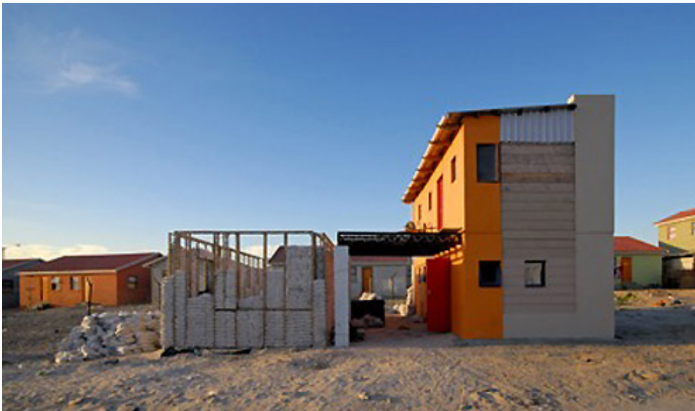
Figure 5.8 : Sandbag Houses a Freedom Park / MMA Architects
