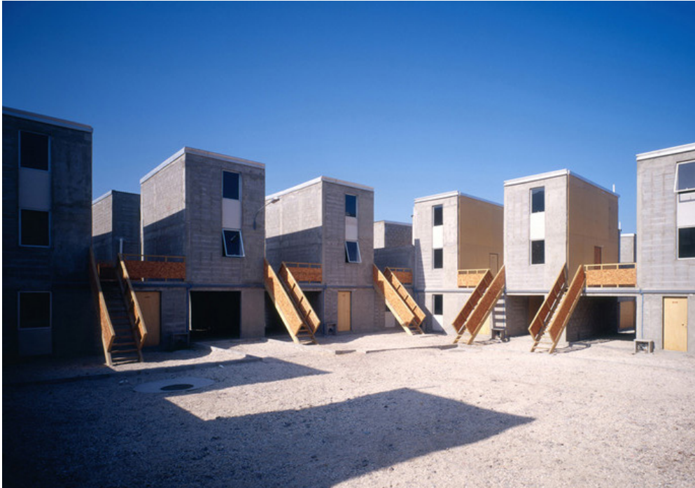
Figure 5.7 : Logements a Quinta Moray / ELEMENTAL
