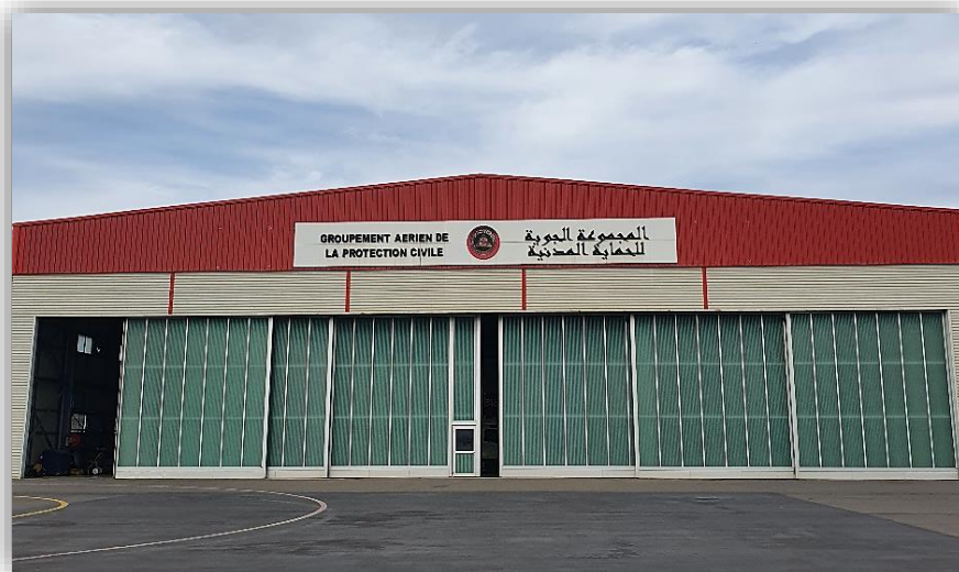
Figure 2.1: The Civil Protection Air Group hangar
