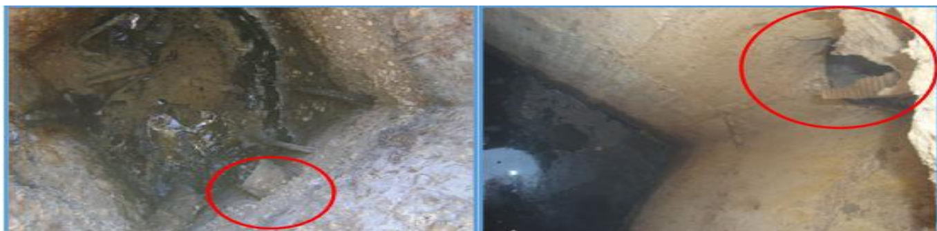
Figure I-4 : branchement irrégulier
