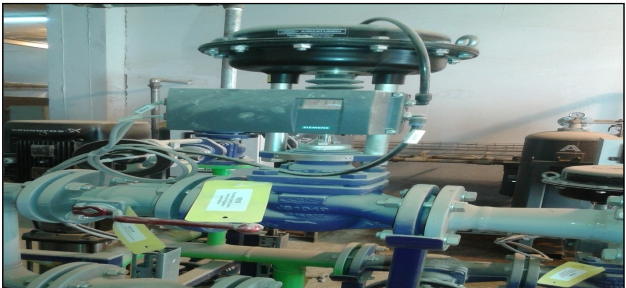
Figure II.1. La vanne proportionnelle
