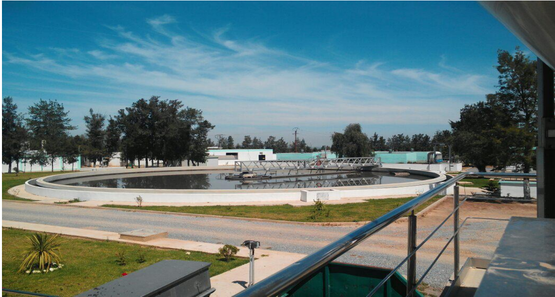
Figure 4. Station d'épuration de Béni Mered (Photo originale)
