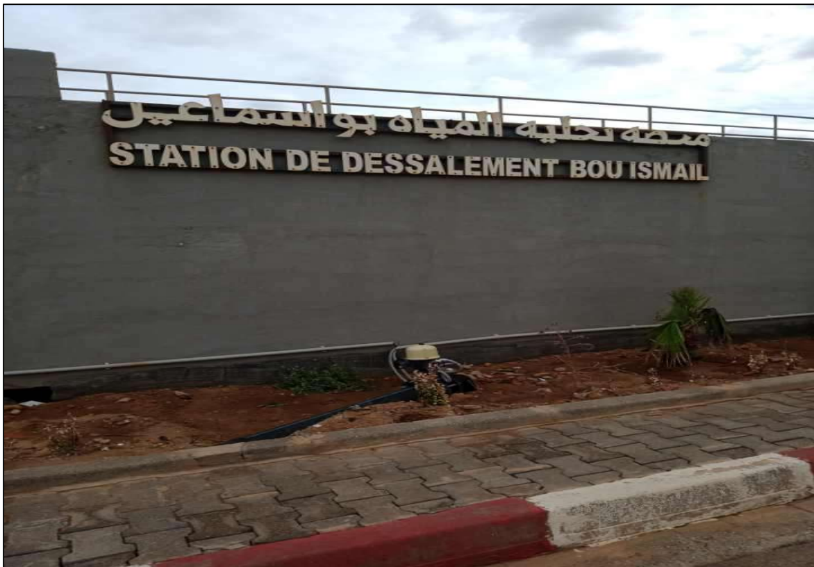
Figure 3. 1 : station de dessalement Bou-smaïl.
