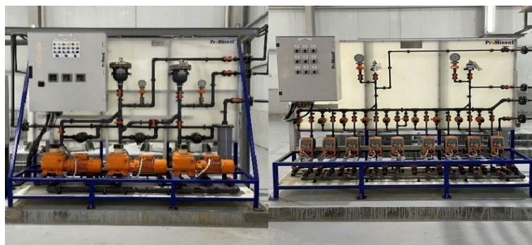
Figure 2.28. Pompes de dosage
