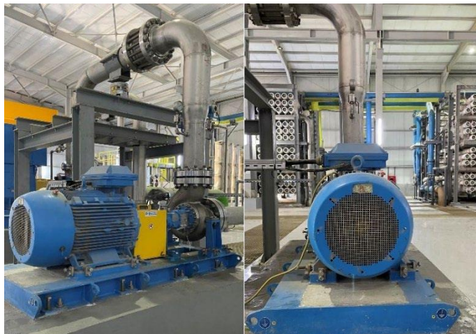
Figure 2.22. Pompes booster
