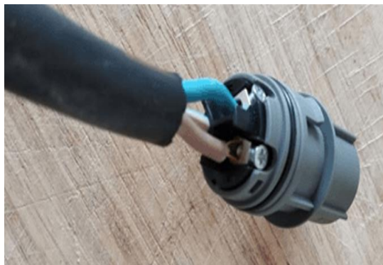
Figure (III.11) : Câbler la lanterne
