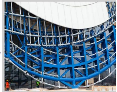
5,500 tons structural steel will carry the outer skin of 40,000 m 2 formed from Fibre Reinforced Plastic (GFRP) panels, a total of almost 17,000 single panels of different geometry
