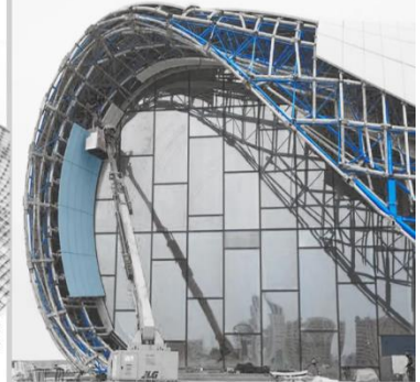
• 121,000 m 3 concrete, 194,000 formwork and 19,000 ton steel forms the RVT
