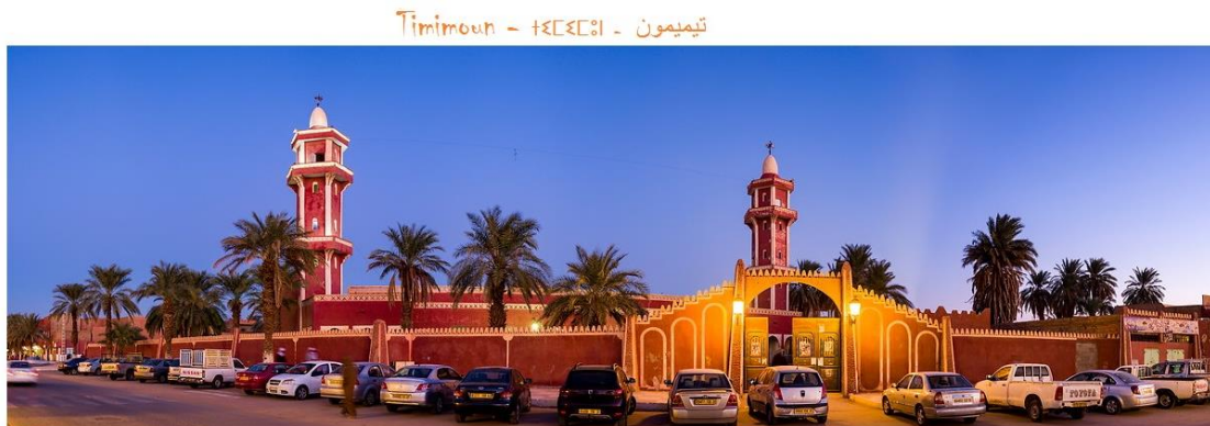
Figure 133: APC de Timimoune ,le style colonial de Timimoune , source : https://www.communesdalgerie.com/
