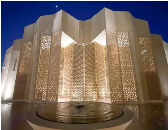
Figure 36 Mosquée de Masdar City, source : Masdar City: The eco-oasis blueprint for sustainable cities | PwC
